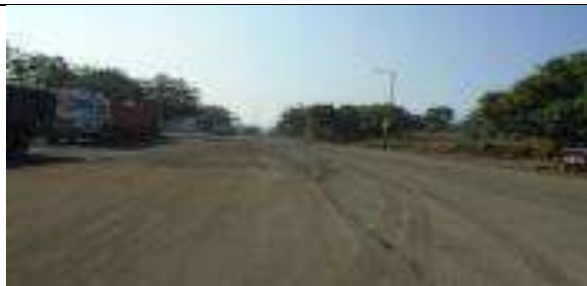
Way to CHP
