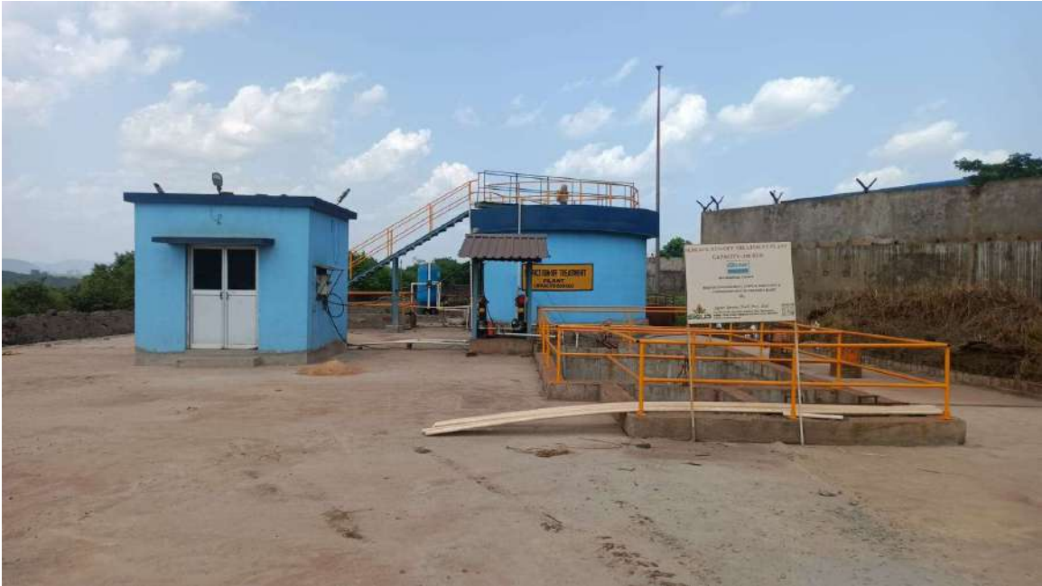
(SRTS – 2: FAP & Briquetting Plant)
