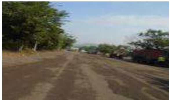
Way to Main-Gate
