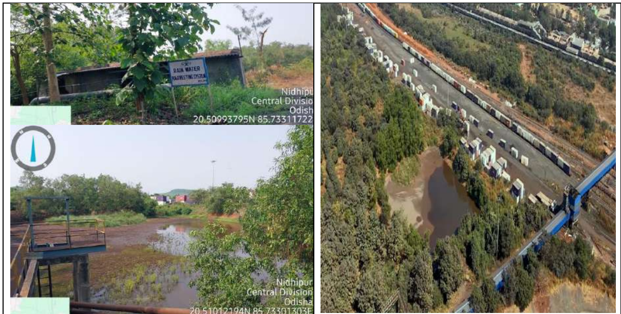
Figure: 11 (Rain Water Harvesting Pond)
