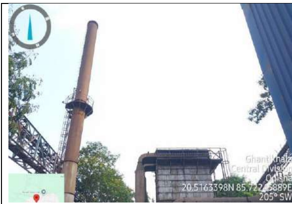
SMS Lime (Stack & Baghouse)
