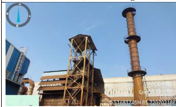
SMS Primary (Stack & Baghouse)
