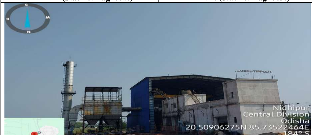
Wagon Tippler (Stack & Baghouse)
