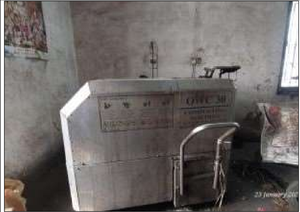
Near Canteen Area
