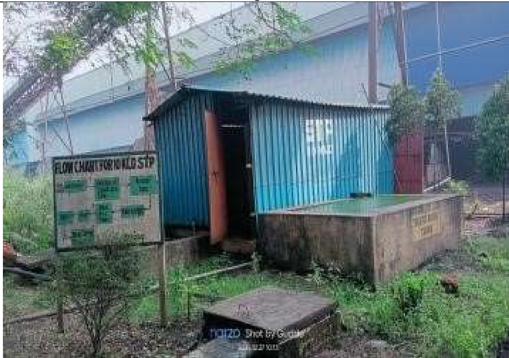
STP 4 – Canteen – 10 KLD
