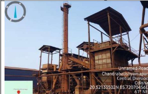
Briquetting dryer (Stack & Baghouse)
