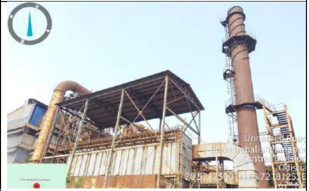
FAP 2x9MVA (Stack & Baghouse)
