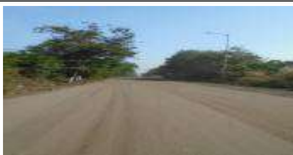
Way to Power Plant
